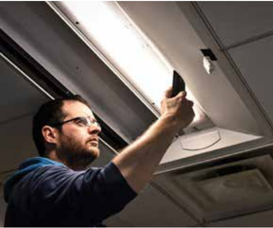
An installer uses a cell phone to configure the system. All but two of the systems ultimately required factory assistance during installation or following setup.
